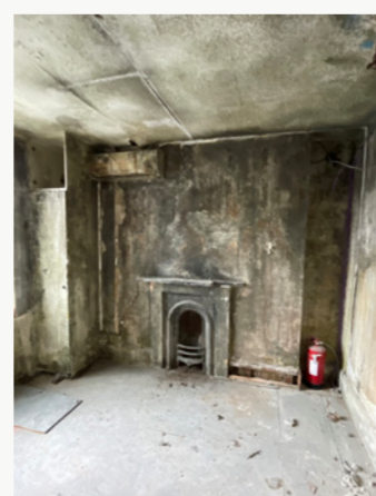
Historic fireplace, some joinery, lath and plaster and floorboards.
