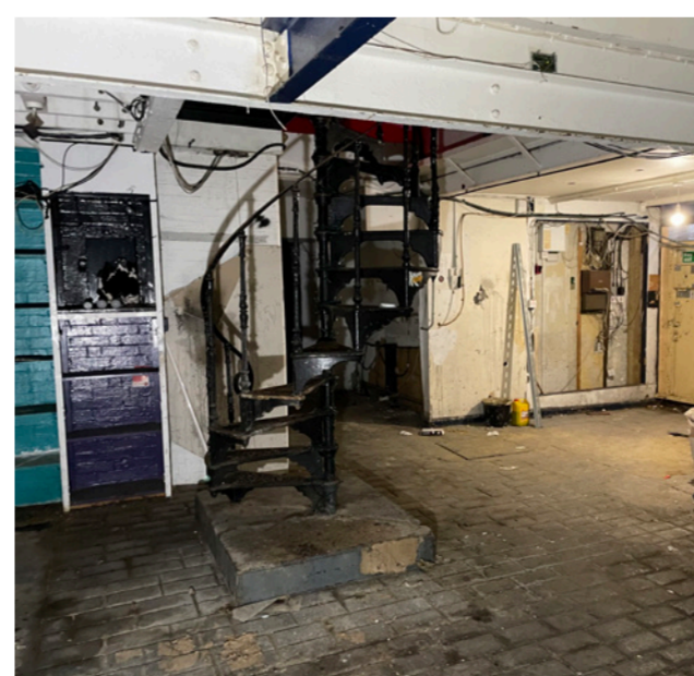
Existing cast iron staircase
