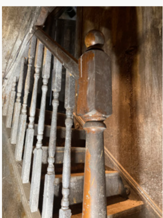
Modern balustrading, treads, risers and stringers cladding.
