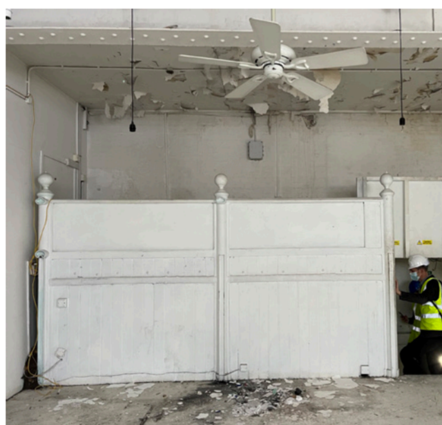
Existing timber horse stalls
