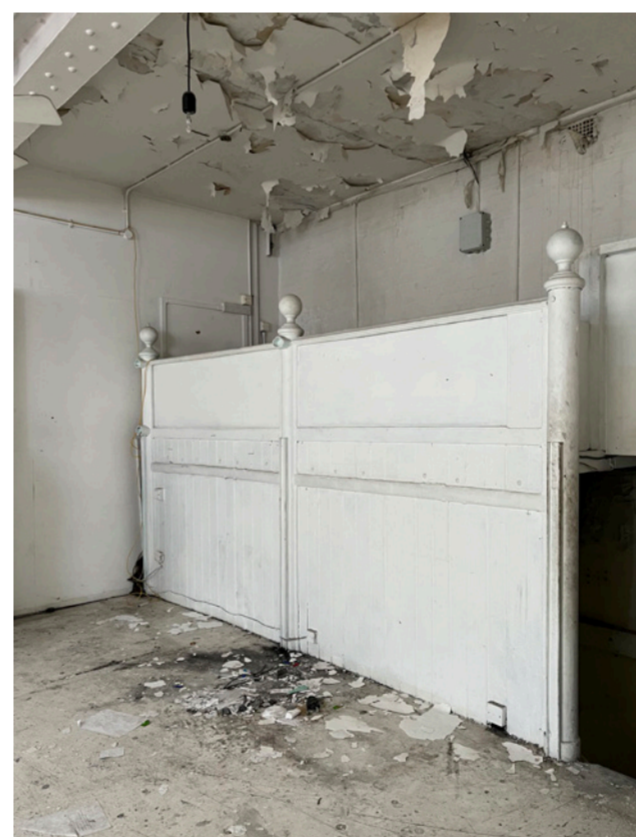
Existing timber horse stalls
